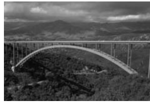
Steel Cold Spring Bridge USA, 1963
