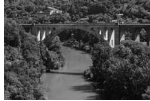
Stone Solkan Bridge Slovenia, 1906
