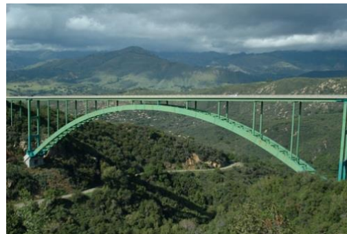
Cold Spring Bridge, USA 1963 Steel 210/371m
