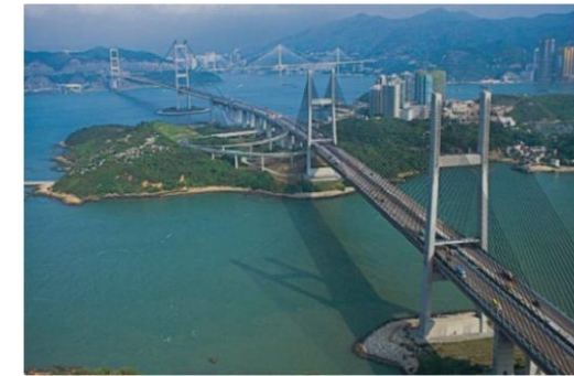
Tsing Ma Bridge, Hong Kong 1997 Steel 1377/2160m
