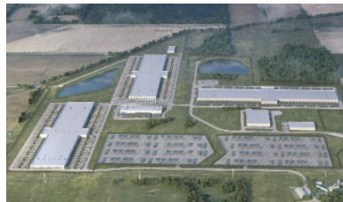
OpenAI, Ann Arbor, Michigan, 1GW, under construction
