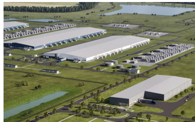
Meta, Lebanon, Indiana, 1GW, under construction
